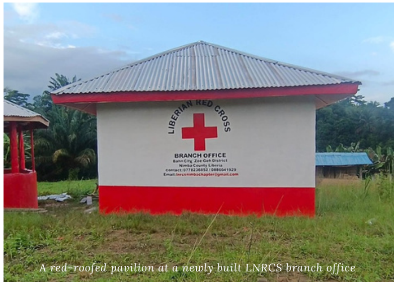
Newly constructed LNRCS branch office buildings in Ownesgroves, Grand Bassa County.
